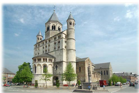
East view of the monastery
